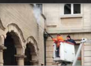
Facade cleaning: without chemicals and damage
